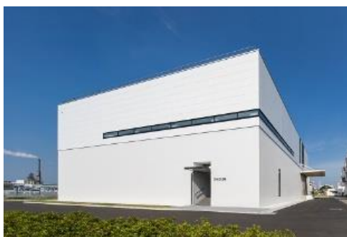
Drug research facility “CRADLE Building”
